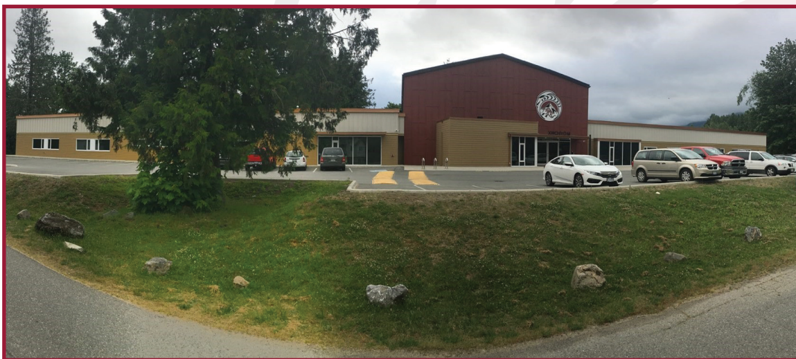
Cheam Health Building
